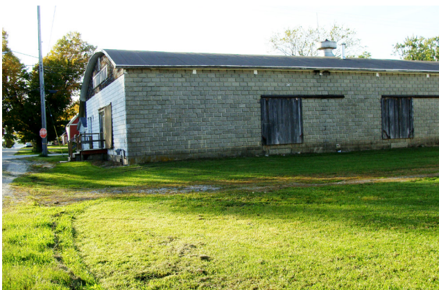
Industrial land use in Lake City area.
